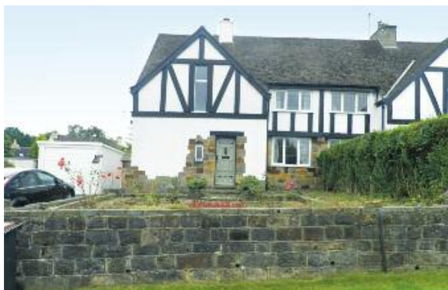
Spring Lane, Burn Bridge
